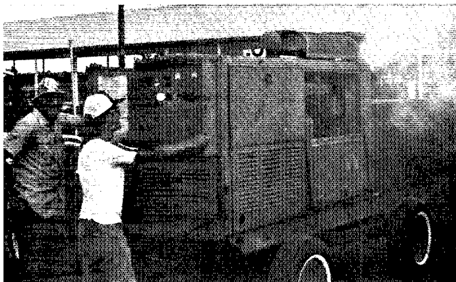
The Tidelands ARS call their generator a "power source and mosquito fogger" (note exhaust smoke at upper right of photo). That sucker looks big enough to supply the electricity needs for a small town. K5YYD and WB5QXZ tend the beast for the K5CA/5 (5A) 1978 Field Day effort.
