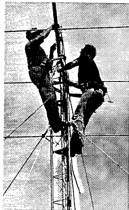
W7GPW (I) and K7YR, putting up the first of two five-element Yagis for 10 phone. The Mike and Key ARC, K7LED/7, 7A.
