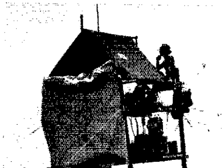
Completed operating stand. Wooden operating stand supported by a couple of guy wires. The upper platform for operation and lower portion was used for generators and gas. JF11ST had one 1.2-kW, one 800-W and two 300-W generators.
