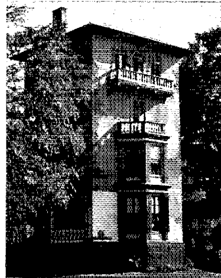
This house, on an estate on the east bank of the Hudson River, was the home of Samuel F. B. Morse from 1847 until his death in 1872.
