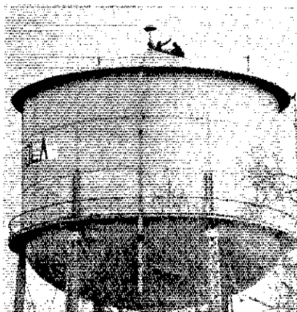
WA0SOF and WB0SXJ top off the Paola, Kansas water tower with the receive antenna for WA0SOF/RPT. The repeater is operated by the Miami County ARC for use during severe weather and tornado watches. The transmitter installation is located a half mile away on the Miami County Sheriff's Department radio tower. The split sites are interconnected via a telephone line. (photo by Gary Ford, WB0UYB)
