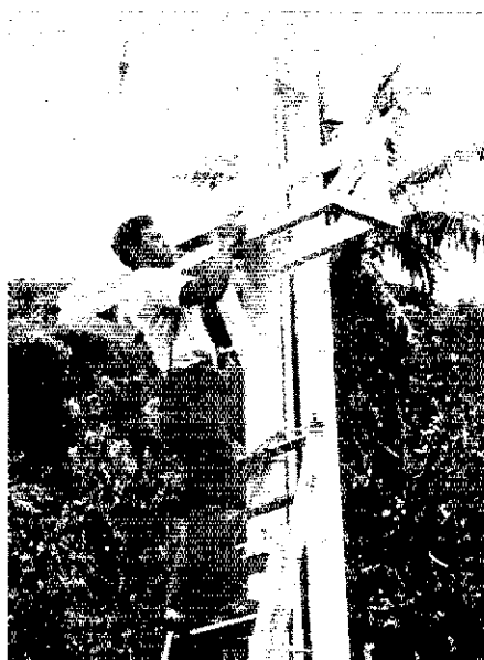
Tom Christian, VR6TC, adjusts a solar-power module on his Pitcairn Island antenna tower. The solar assembly is an alternative power source to the island's costly diesel-powered generator. (photo courtesy Motorola, Inc.)
