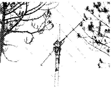
The mast-to-pipe U bolts are loosened and the boom is turned to a horizontal position. This puts the elements in a vertical plane. Then, the pipe U bolts are tightened and pinning bolts secured. The boom U bolts are then loosened and the boom turned axially 90°.
