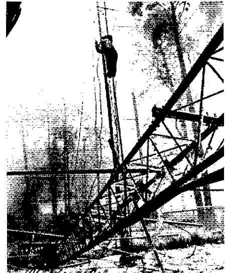
This is the wreckage of the tower holding the Birmingham Amateur Radio Club repeater, W4CUE/R, after a tree fell across the guy lines. WA4JUM (on the tower) was one of a crew of volunteers who put W4CUE/R back on the air. (photo courtesy of N4DMA)
