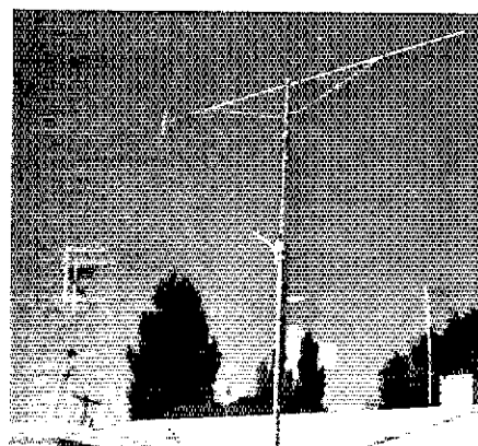
W5RKS keeps the bands hopping from New Mexico with a single, 19-element Boomer at 30 feet on 144 MHz and four 8-element quagi antennas for 432.
