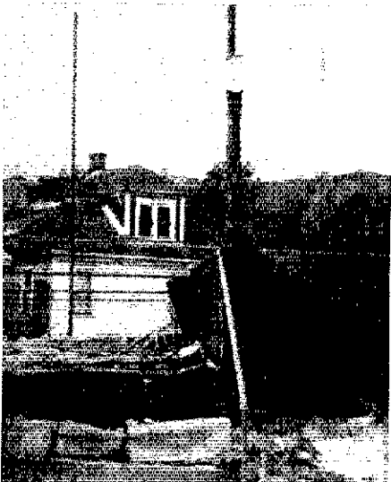
Like the Phoenix, the bird of mythology rising out of the ashes, what appears to be a Wouff Hong looms above the remains of a house. Art Mueller, W3BKD, of McDonald, Pennsylvania, took this photo while traveling through the town of Slovan.
