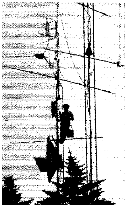
WA2AAU putting the finishing touches on W2SZ's 35-foot rotating tower, which allows their microwave antennas to be pointed to within a half-degree.
