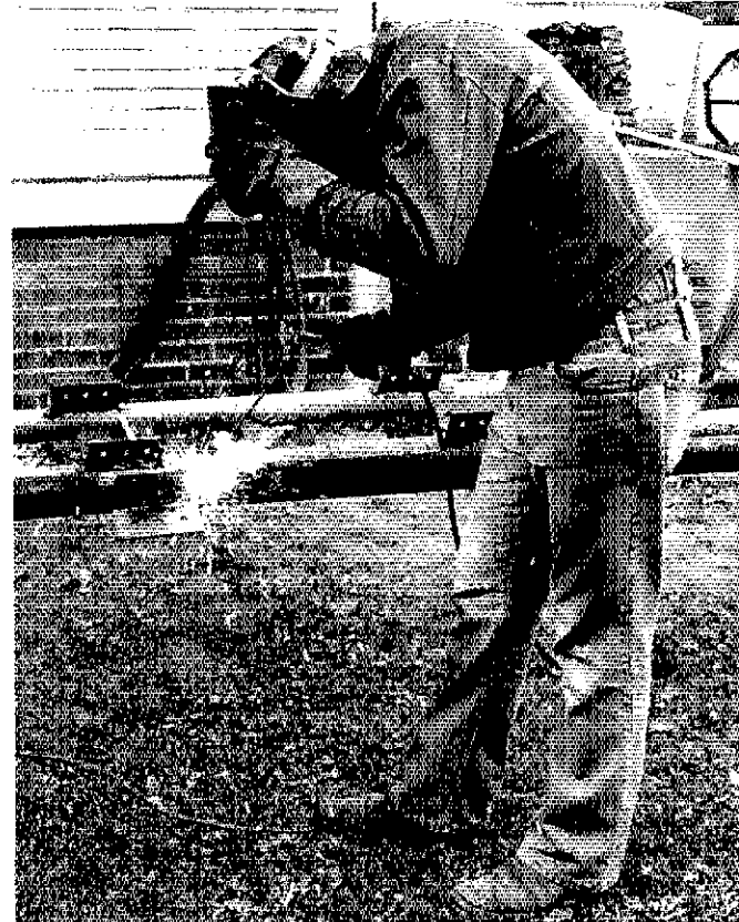
Fig 5—John Baublitz, WD8RXP, welds plates to upper tower leg sections.
