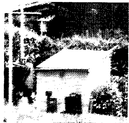
Fig 4—All fuel is stored in an isolated aluminum shed. This shed is near the rear of my lot, and far from the house and power shed. (You caught me leaving the cans out!)
