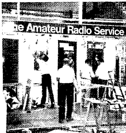
The TELECOM-87 Amateur Radio Stand under construction. . . .
