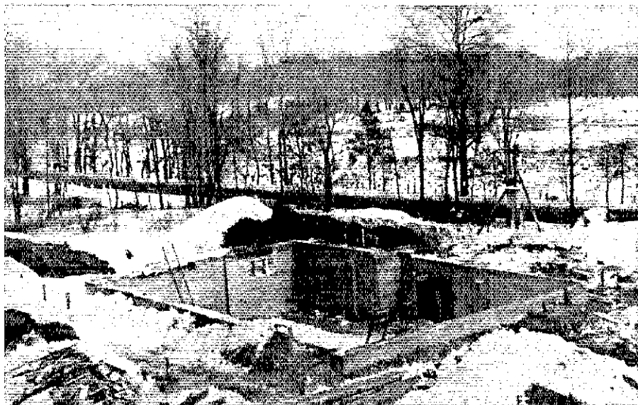
It was a long, cold winter, but work continued on the new building into early 1938.
