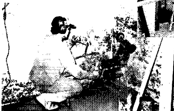
A concrete worker bores holes in the existing foundation for new antenna lead routing.
