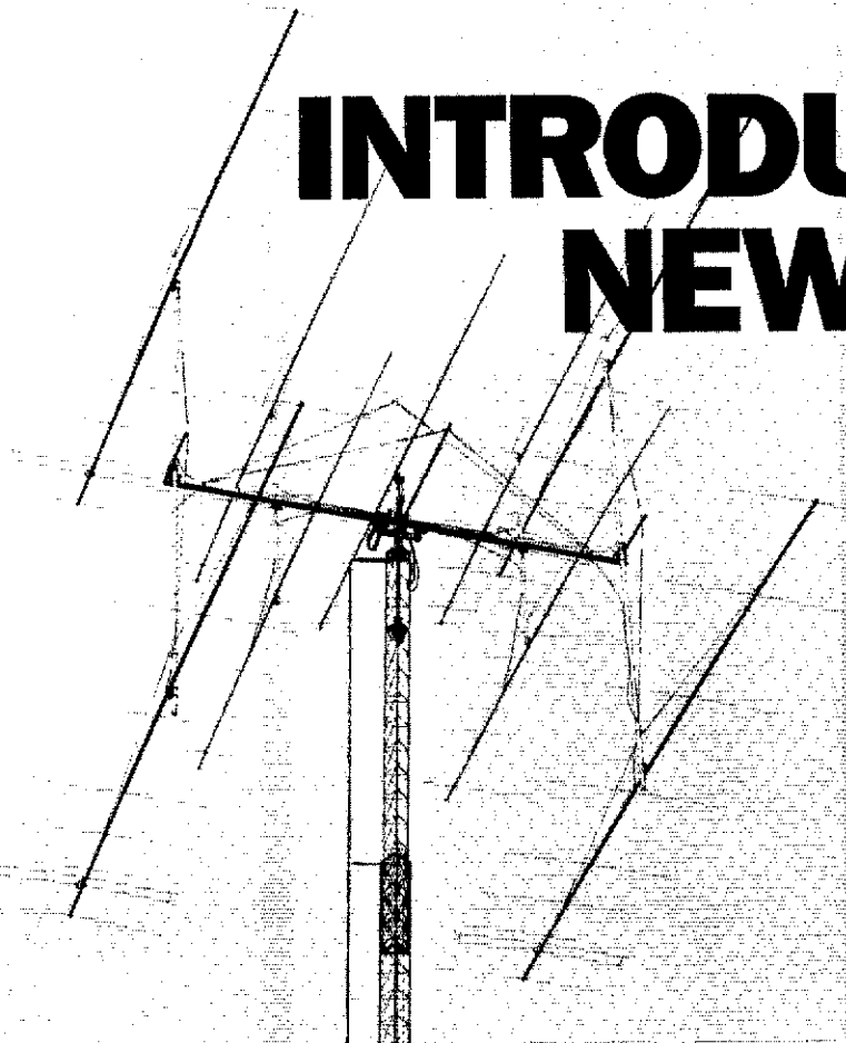
6-meter and 2-meter moonbounce installation. Four 6M-2WL, four 2M-5WL and one 432-13WL antennas in array on self-supporting 89-foot US tower at N7ML.
