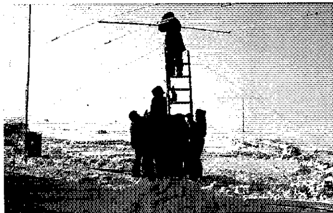
Installing a beam in frigid arctic air is a true team effort. (photo W6MKB)
