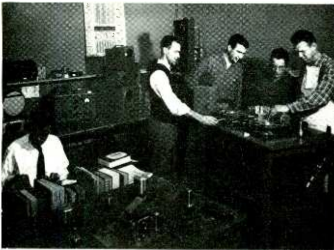
The photograph shows five of the original group working with an arcuate head scanning system which was eventually abandoned in favour of the transverse scan arrangement. Block diagram on the right was the first of a complete system using transverse heads, modulation-demodulation and sequential switching. Unlike present machines, heads were ganged in tandem, and 300 rps used as the drum speed.
