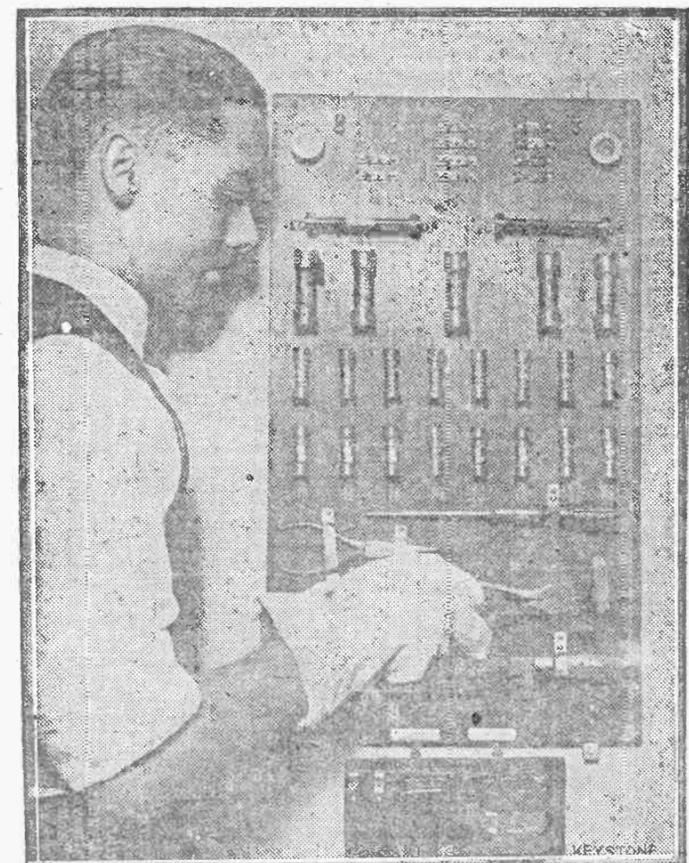
WEAF (New York city) probably has the first radio "first aid" kit in existence. Handily placed, it contains fuses, choke coils, grid leaks, as well as the ever useful pliers, wrenches, etc., and a small buzzer tester. It is a handy article in "shooting" and remedying sudden breaks and is one of the reasons WEAF is always on the job. Photo shows the kit at the Walker street, New York city, station.
