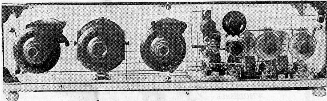
Here are top and front views of the famous Superduc Deluxe. A glass cabinet was used because it allowed the parts and their arrangement to be shown with utmost clarity. As stated in the article, the only advantage in a glass outfit is in its appearance.
