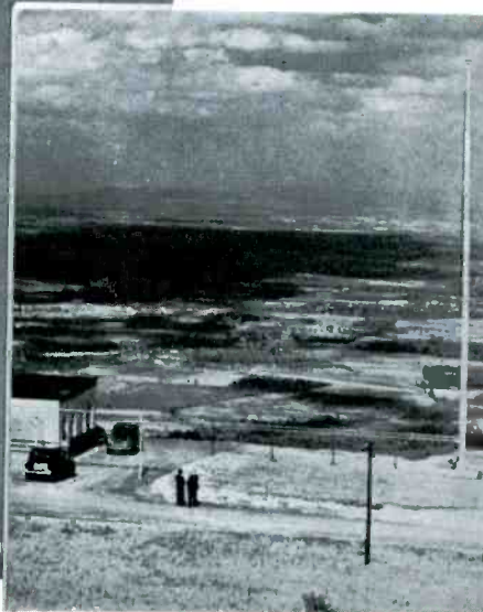
FIG. 4. CLOSE-UP OF THE ANTENNA USED AT THE HELDERBERG STATION FOR TESTING THE 50-KW. TRANSMITTER, AND A VIEW FROM THE STATION OF THE VALLEY BELOW
