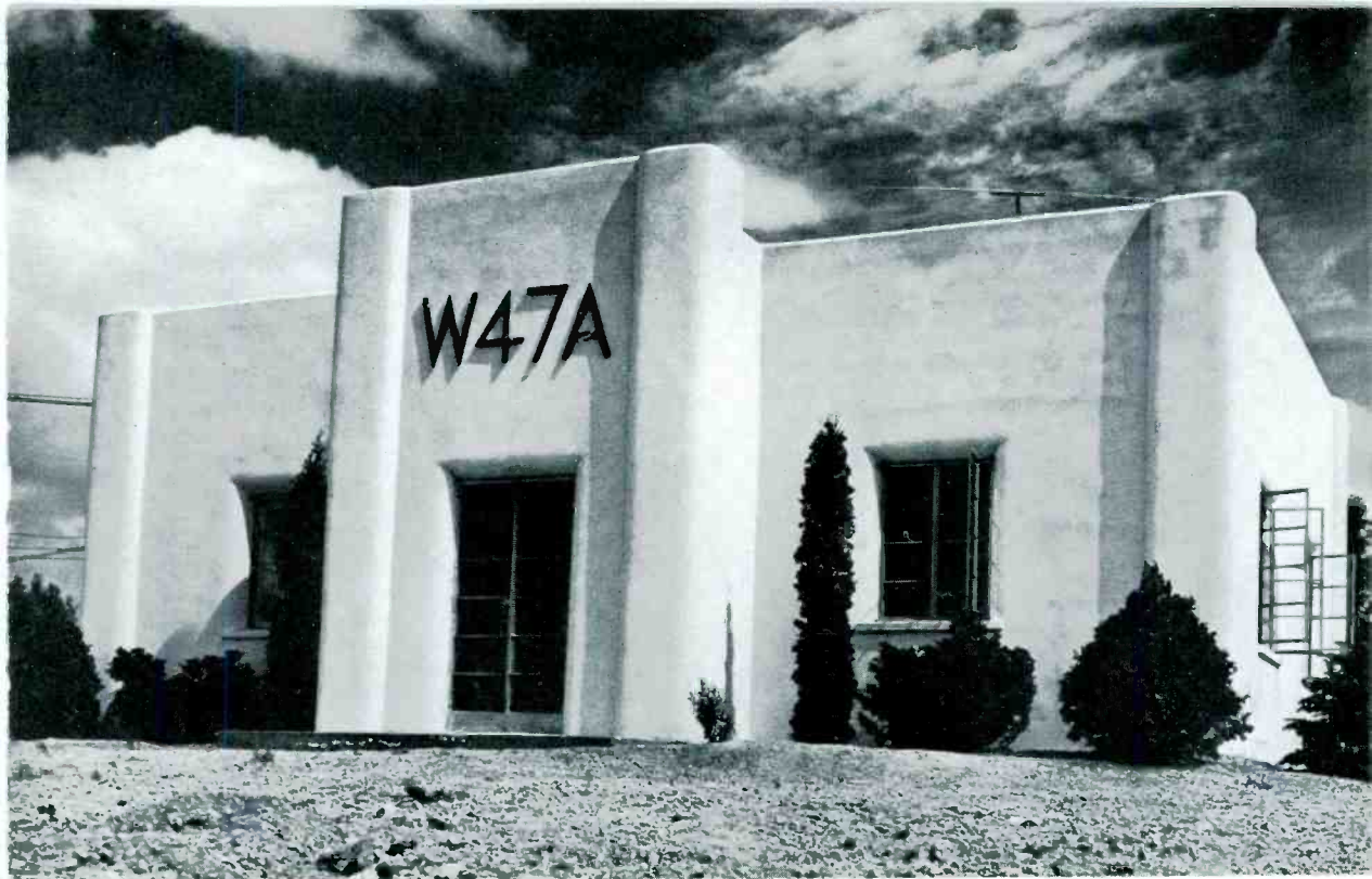
W47A TRANSMITTER HOUSE TOPS MT. PINNACLE, 1,600 FT. HIGH, NEAR ALBANY, N. Y.
