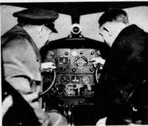
High over Boeing Field in Seattle, aviators test the automatic control which guides a plane in response to pressure on buttons. Human pilots are needed only to land the plane.
