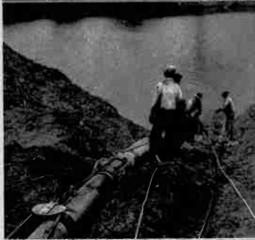
Snaking the pipe line across the Minnesota river near Minneapolis. Tractors pull the closed-off pipe through the water with long chains and cables.
