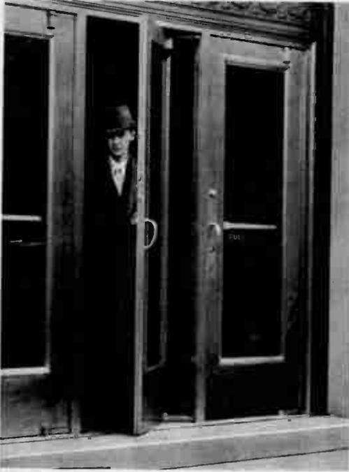
These bronze doors, installed at Kanawha Valley Bank in Charleston, West Virginia, pivot inward when pushed out, as shown. Compression springs on pivot arms close door.
