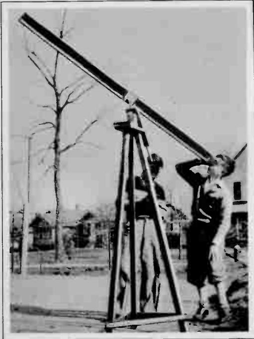
This simple equatorial telescope mounting, built by 14 year old Iowa youth, costs less than \$5 including good grade lenses. Tripod stand is made of 2"x2" pine lumber.
