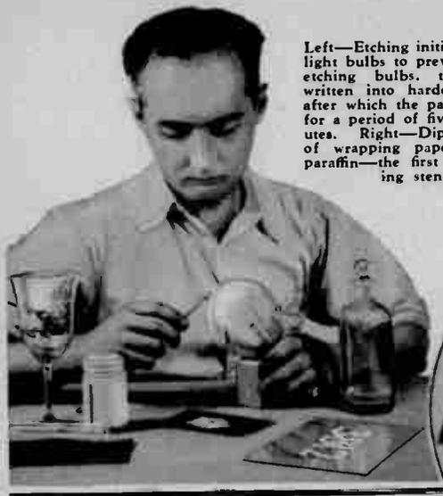
Left—Etching initials on electric light bulbs to prevent theft. In etching bulbs, the name is written into hardened paraffin, after which the paste is applied for a period of five or ten minutes. Right—Dipping a piece of wrapping paper in melted paraffin—the first step in making stencils.
