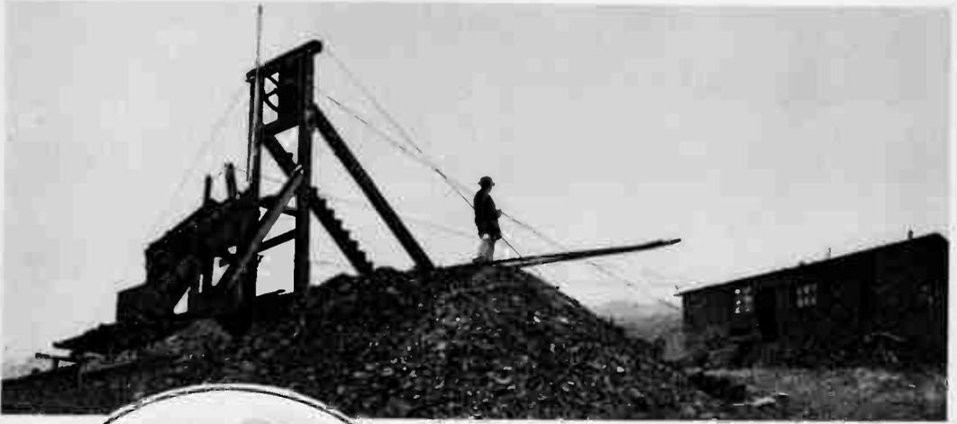
A general photo of the mine showing the scaffold, the shaft head, and the power house. The power house was built from salvaged lumber and houses the power plant constructed from the chassis and motor of an old Dodge automobile.
