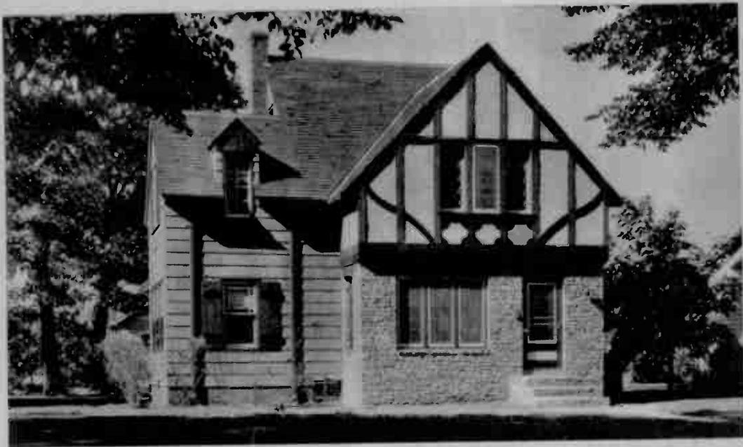
Lower right—A semi-bungalow before remodeling. Above—The same bungalow rebuilt into an English type house by adding a front gable, a side addition, shingling the sides, and putting stone work on the "first floor front." The change brought a larger living room, a coat closet, a private porch, a sleeping porch, and a distinctive home exterior for \$3,375.
