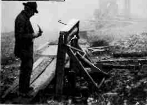
Howard Wheery at the old hand windlass set over the course of the old vein. The junk made scaffold and shaft head rear high into the air in background, as landmarks of success.
