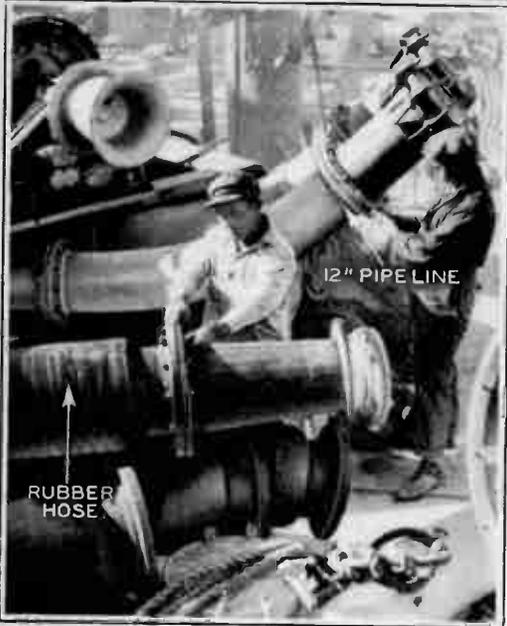
Men on the vessel preparing the filling pipes to receive the rubber hose which is connected to the pipe line from shore.
