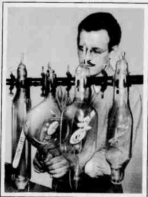
Advertising emblems sealed into these cathode ray tubes glow weirdly under electron bombardment. Gilbert T. Schmidling (pictured above) builds these tubes for store window display. High voltage transformers are needed here.
