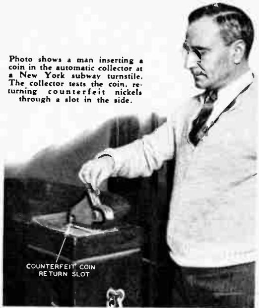
Photo shows a man inserting a coin in the automatic collector at a New York subway turnstile. The collector tests the coin, returning counterfeit nickels through a slot in the side.
