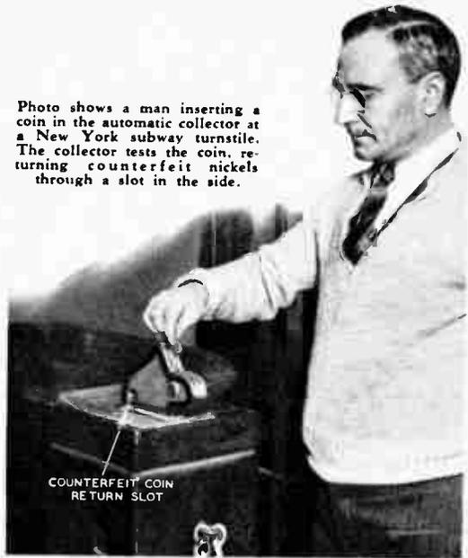
Photo shows a man inserting a coin in the automatic collector at a New York subway turnstile. The collector tests the coin, returning counterfeit nickels through a slot in the side.
