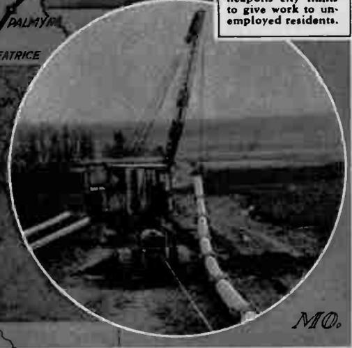
Tractor cranes swung the snake-like pipe line into waiting trenches after crews had joined sections of pipe with flexible couplings. Tractor in foreground is pulling pipe ahead.
