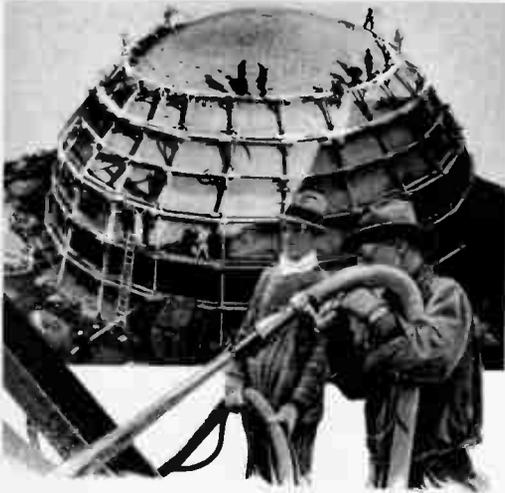
Above—A view of the planetarium dome, erected without costly cement moulds. Inset—A close-up of the mixing and spraying hose used in constructing the huge dome.
