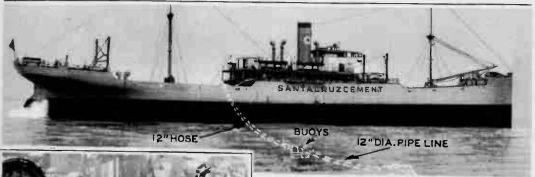
Above photo shows a bulk cement freighter ready for loading. A 12-inch pipe line is floated 2,500 feet to the ship on buoys which support the line over the water's surface.
