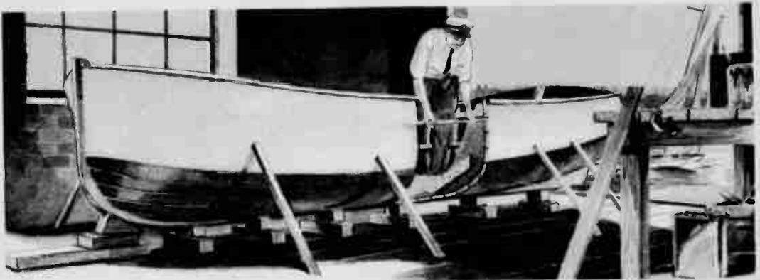
would take the boat's weight in water to fill the hollow. Now if we were able to solidify this water we poured into the hollow, then remove and set it up on a sharp edge as a fulcrum, the point of balance would be the center of buoyancy.
