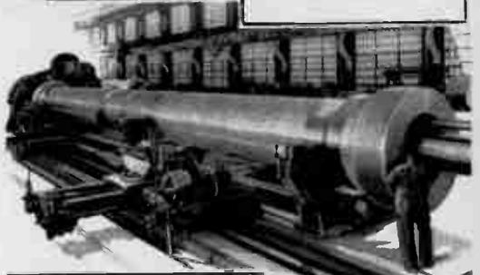
Forged cylinder is machined inside and out before ends are closed in by final forging process. Lathe used is one of the largest in the world.
