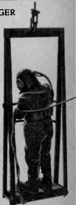
A view taken inside the oval fender showing the metal frame used for lowering the divers into the water and for removing him from the bottom to the surface. Divers were often compelled to work 100 feet under water surveying pier sites.
