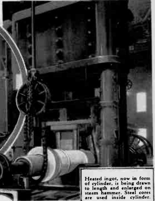
Heated ingot, now in form of cylinder, is being drawn to length and enlarged on steam hammer. Steel cores are used inside cylinder.
