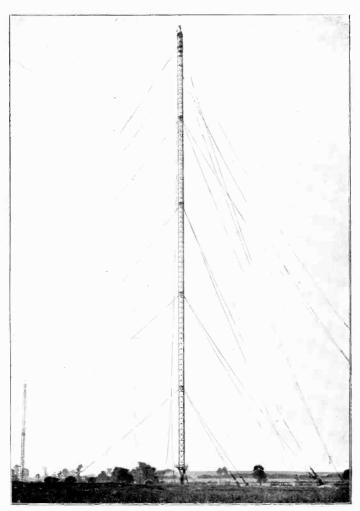
FIG. 1. AN 800-FOOT MAST AT THE RUGBY STATION
