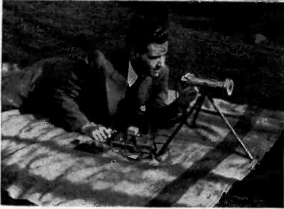
The operator taps out a code message on an ordinary telegraph key. Below he sights along the barrel to aim the flash light
