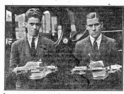
Two large transmitting vacuum tubes which are now on exhibition at Albert Hall, London, England. These are the tubes used at the new Station 5XX, Daventry. They are known as the Holybdenus Electro Valves, have a power of 1 kilowatt, and cost £60.
