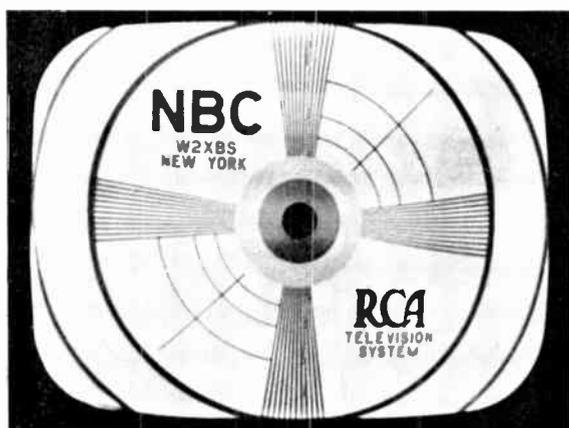
Figure 57—Normal Test Pattern
