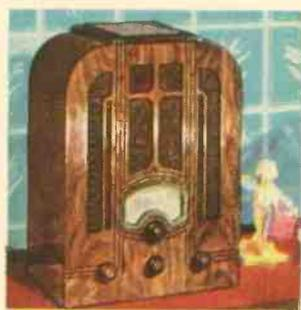
Table Model T6-1. A 6-tube superheterodyne. Tuning range 540 to 18,000 kc. \$49.95.
