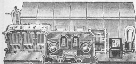
The 1929 Screen Grid Nine Tube Laboratory Receiver is a Super-heterodyne having only two tuning controls for a total of five stages of R. F. Amplification! It is an ultra selective receiver giving positive 10 Kilocycle separation between stations, and capable of 2000 to 3000 mile regular reception range with marvelous tone quality.
