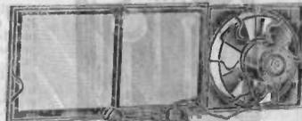
The Electric Portable Ventilating Fan is quickly and easily installed in any window. It is adjustable to varying widths. A great health producer at a moderate price. Changes the air every four minutes in the average hot kitchen, stuffy living room, smoky den, or oppressive bedroom. Very economical to operate. Costs four cents for twenty-four hours' service. The attractive panel is made of 22-gauge steel and will not warp. Glass panel may be obtained at a small additional cost.
