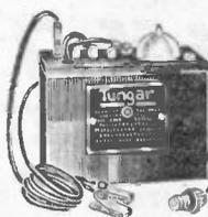
Made by the General Electric Co. Charges 6 or 4-volt batteries at 1/2 amp. rate.
