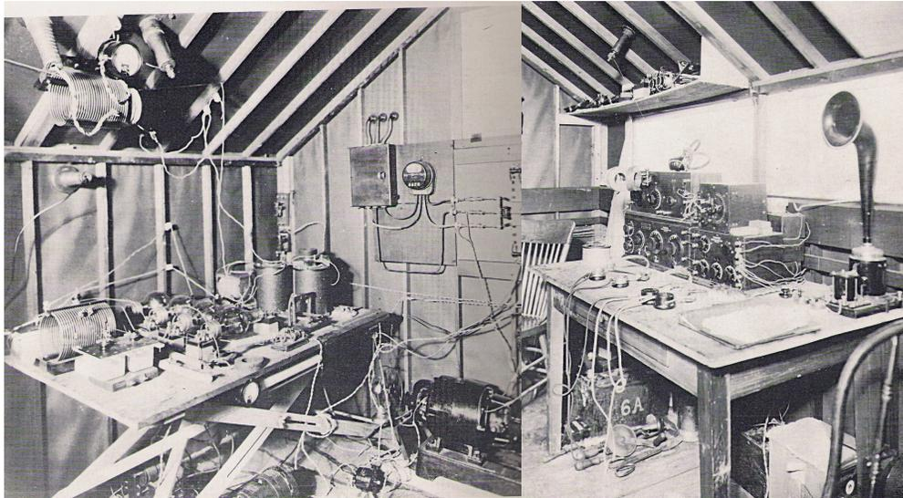
**Figure 3** Picture on the left, the IBCG transmitter, employing four type “P” Radiotron UV204 vacuum tubes, the oscillator tube on the right, the three tube amplifier on the left. A 2000 volt DC motor generator provided the HV power supply. The receiver, on the right, on the opposite side of the shack, employed the Paragon RA 10, a superhetrodyne regenerative receiver, and a BFO circuit for CW reception.
