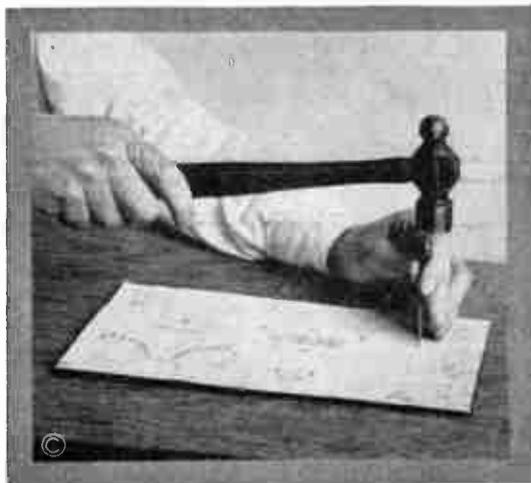
Plate No. 3—Marking panel from Template
