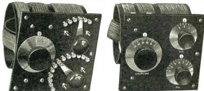
6A9663—Vario Coupler Unit, With Switches Front Mounted.
