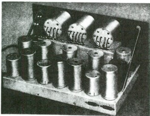
Front view of new "AGS" commercial or "pro" type short wave receiver, with "single dial" control. Yes, it's a super-het!
