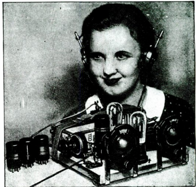
The "Globe-Trotter" in actual operation, with extra plug-in coils at the left.
