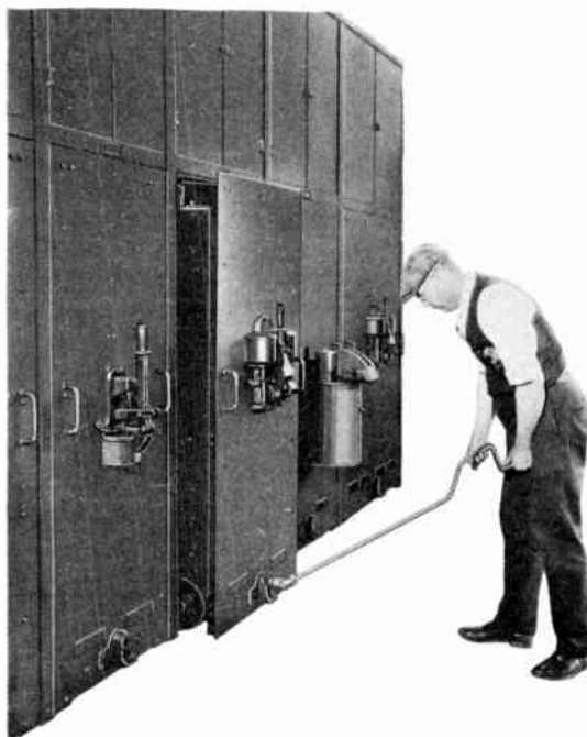
Fig. 127. Method of Inserting Truck with the Cranking Handle
