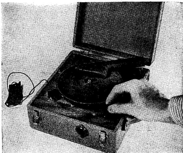
Assembled portable radio phonograph, showing 6" turntable, volume control knobs, and dial
