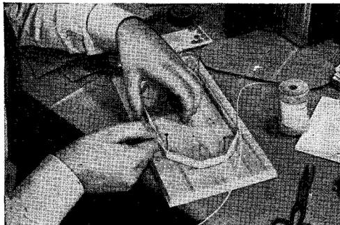
**2** Remove the cardboard, and wind either No. 24 or No. 26 double-cotton covered wire around the nails in the form. Approximately 50 turns will be needed. Wind the wire evenly and tight
