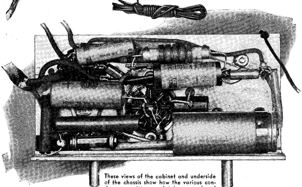
These views of the cabinet and underside of the chassis show how the various condensers, resistors, and tubes are placed
