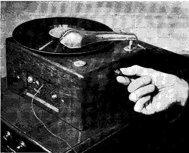
Plugged into an outlet anywhere in the room with your radio, the unit "broadcasts" records through the loudspeaker
