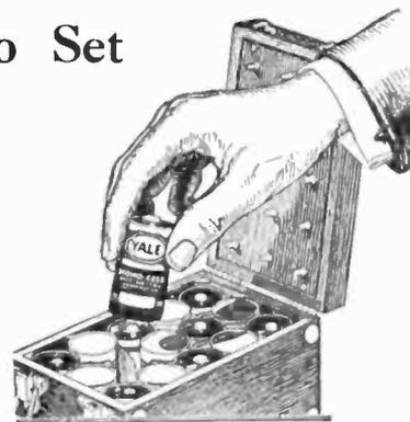
The Yale Mono-Series Radio B Battery allows instant replacement of any under-voltage cell. Standard Yale Mono-Cells are used—procurable everywhere. Fifteen spring contact points assure positive connection. A five point switch allows 16½-22½ volts variation. Dark walnut finish wood case. Hard rubber binding posts.
