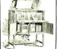
All parts of tone chamber, set compartment and battery space perfectly accessible. The A battery sets on leaf which pulls forward for easy filling or testing
