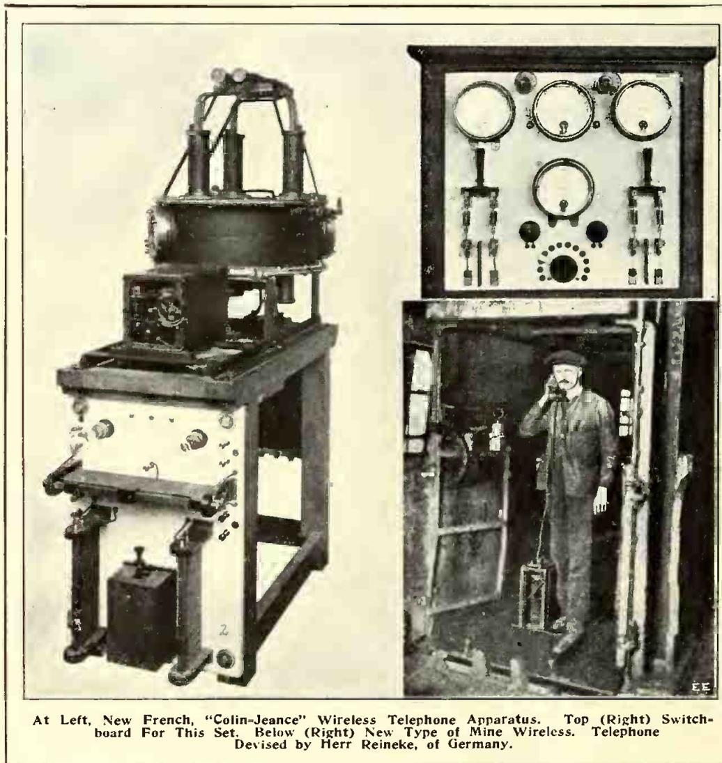
At Left, New French, "Colin-Jeance" Wireless Telephone Apparatus. Top (Right) Switchboard For This Set. Below (Right) New Type of Mine Wireless Telephone Devised by Herr Reineke, of Germany.
