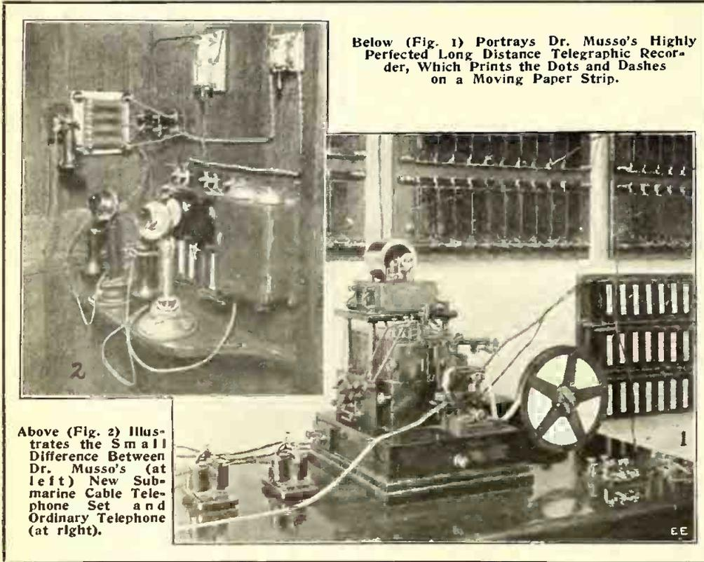
Below (Fig. 1) Portrays Dr. Musso's Highly Perfected Long Distance Telegraphic Recorder, Which Prints the Dots and Dashes on a Moving Paper Strip.
