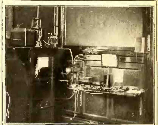
Wireless Set Used to Extend Operation and Usefulness of Regular Telephone System.
