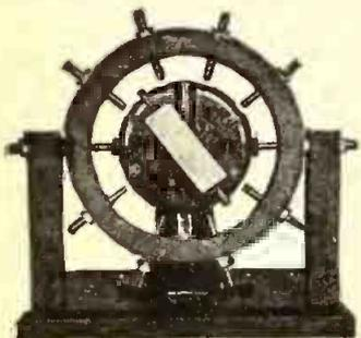
Gives 600 cycle whistling spark like a quenched gap. Attains full speed in 1 second; stops dead inside of 3 seconds. You do not have to wait for this rotary to start nor do you have to wait for it to stop. It always beats you to it. The light revolving discharge arm allows a quick start and quick stop. Will work on sets up to 1 K. W. Used on 60-cycle current.
