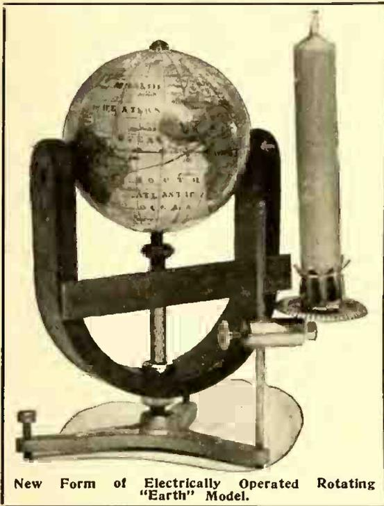
delicately mounted between the poles of a strong permanent steel magnet C, as the illustration shows. The sphere measures 2½ inches in diameter, but this may be varied somewhat in case the experimenter intends building one.
