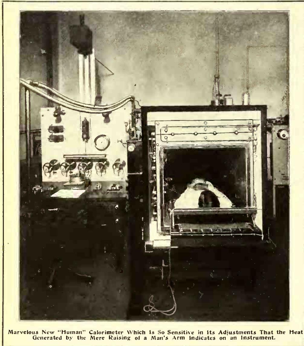
Marvelous New "Human" Calorimeter Which Is So Sensitive in Its Adjustments That the Heat Generated by the Mere Raising of a Man's Arm Indicates on an Instrument.
