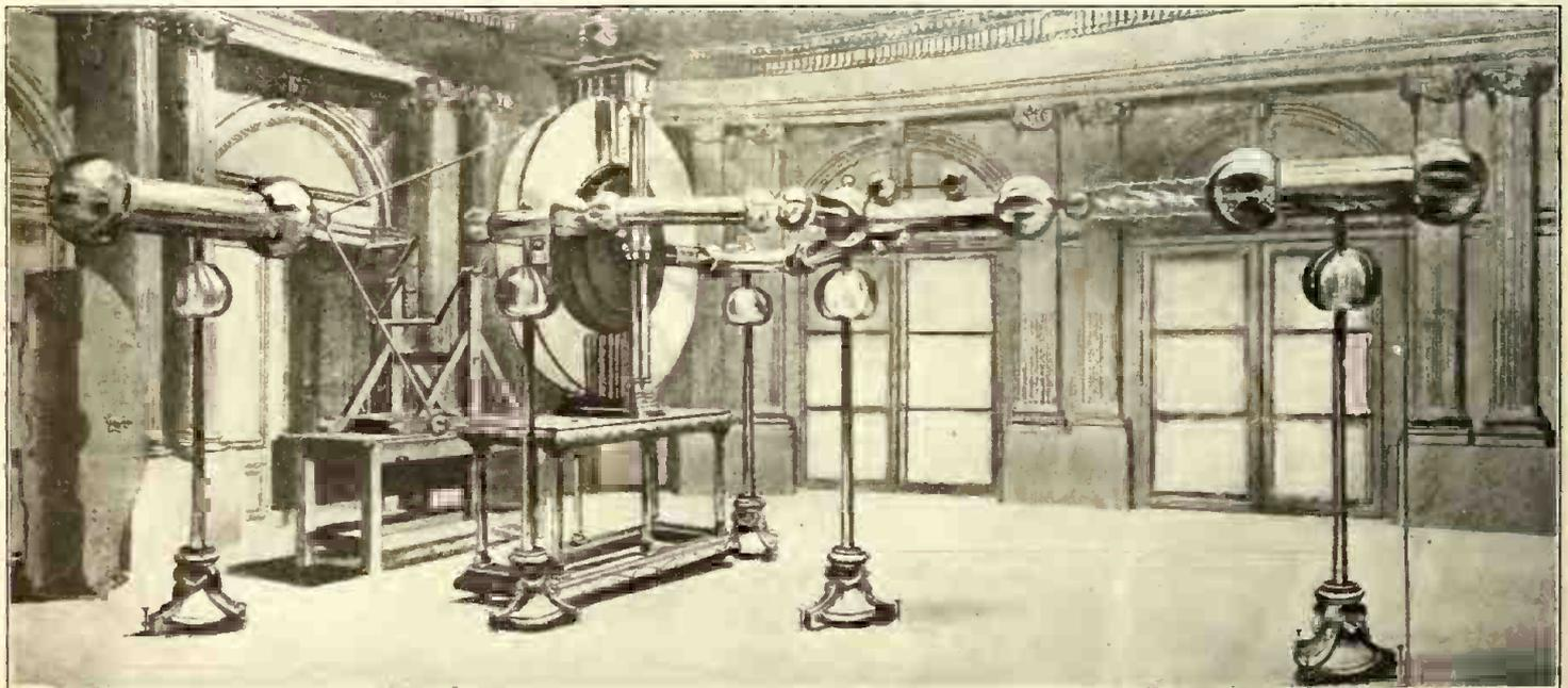
Fig. 3. This Portrays an Early Static Machine of Massive Proportions, Built in 1785 by Martinus Van Marum. This Ponderous Machine Standing 10 Feet High, Produced But 8-inch Sparks.
