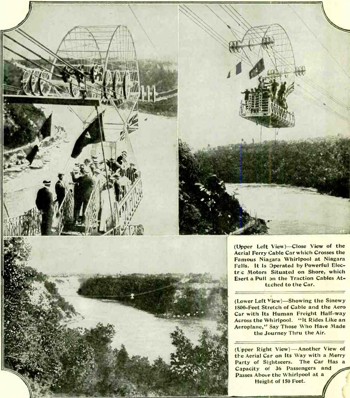
(Upper Left View)—Close View of the Aerial Ferry Cable Car which Crosses the Famous Niagara Whirlpool at Niagara Falls. It is Operated by Powerful Electric Motors Situated on Shore, which Exert a Pull on the Traction Cables Attached to the Car.
