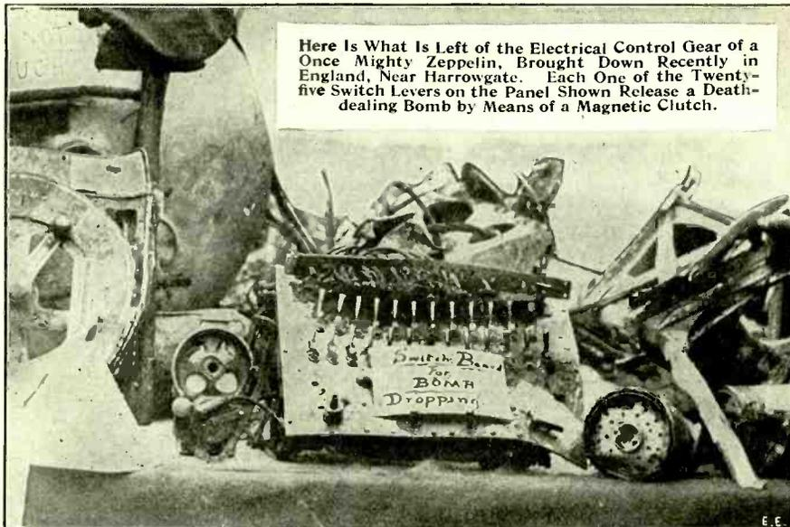
Here is What is Left of the Electrical Control Gear of a Once Mighty Zeppelin, Brought Down Recently in England, Near Harrogate. Each One of the Twenty-five Switch Levers on the Panel Shown Release a Death-dealing Bomb by Means of a Magnetic Clutch.
