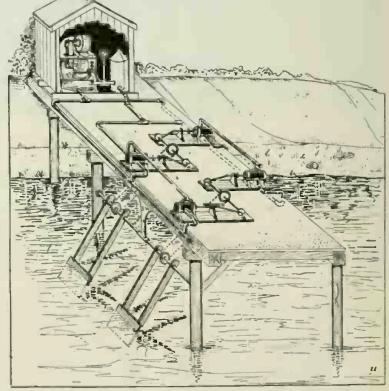
Fig. 3—Perspective View of New Hydraulic Transmission and Regulation Type of Wave Motor installed At Long Beach, California.
