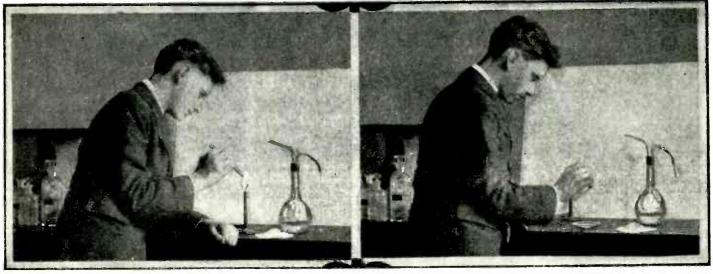
Left—Caution Must Be Exercised Here When Making the Preliminary Tesks Where a Substance Is Heated in a Closed Tube. Right—Treating for Chloric Acid by Cautiously Dropping a Bit of the Substance into a Watch Glass Containing 2 C.C. of Concentrated Sulphuric Acid.
