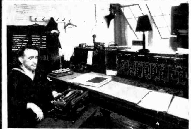
In the left background of the above photo may be seen the switchboard connecting with various points along the Atlantic coast. On the right hand side of the picture are the relays and keys used in connection with these lines.
