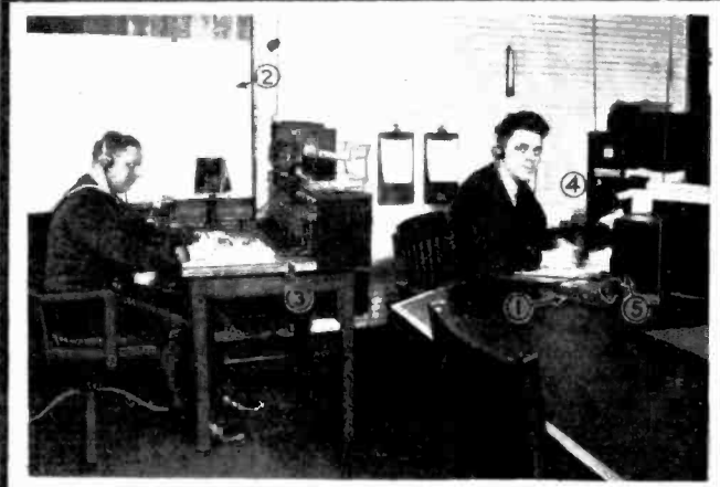
A view of one corner of the operating room is shown above. 1 indicates the keys used to control the transmitter shown in the upper right hand corner, 2 the compass chart, 3 the keys communicating with the compass stations, and 4 and 5 receiving sets tuned to 900 and 600 meters respectively.
