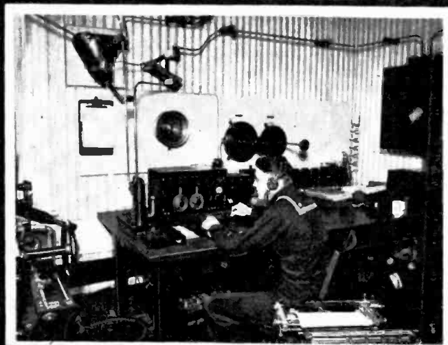
The receiving set situated in the transmitter room is shown herewith. The motor-generators are controlled by a switch on the lower left hand corner of the table. The wheel controlling the wave changing switch can be seen at the left hand side of the photo.
