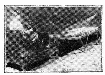
The above photograph shows the new mechanical device which helps to instruct one in driving a car. The picture was taken at the Dresden exhibition.
