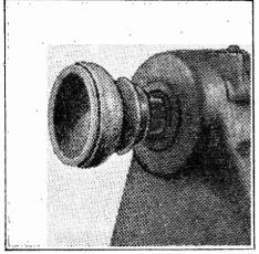
After turning the lid on the inside, turn the box complete, as shown; at which stage it is ready for chucking the lid.
