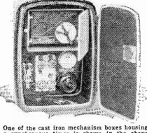
One of the cast iron mechanism boxes housing a synchronous timer is shown in the above photograph.
