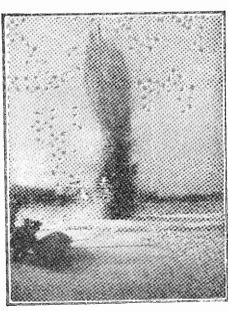
A terrific explosion takes place when thermit is used to crack and break up ice jams. In this case the thermit can was shot high in the air, and the whole ice sheet was lifted and ruptured.
