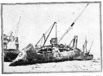
The above photograph shows the German battle cruiser Moltke, which was raised from the bottom at Scapa Flow, Scotland, where it had been sunk after the war. The two air locks may be seen attached to the bottom of the hull. The cruiser was refloated largely through the agency of compressed air.
