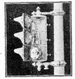
Above is a photograph of a three-color one-way vertical bracket type of traffic signal, mounted upon a short arm bracket. The doors of the signal have been left open.
