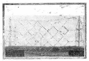
At the left is a photograph of the double projecting antenna erected at St. Assise for radio telephonic transmission toward Algiers. This combination antenna-projector is formed by a metallic trellis stretched vertically between two supports about twenty feet high, the sides of the meshes being equat to one-half the wavelength. Short-waves, 30 meters in length, are used for communication.
