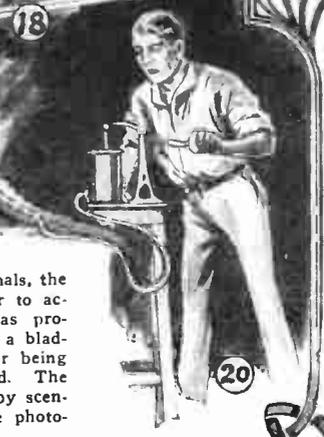
In close-ups of some of the animals, the audience could see them appear to actually breathe. This effect was produced by means of a pump and a bladder as shown above, the bladder being rhythmically inflated and deflated. The rubber tube was either hidden by scenery or else not included in the photograph as in Fig. 18.
