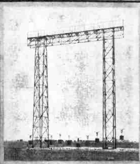
Towering nearly 500 feet into the clouds, the splendidly designed masts support the antenna by a system of counterweights which allows for the expansion and contraction of the wires due to temperature change. The masts are of steel construction throughout.
