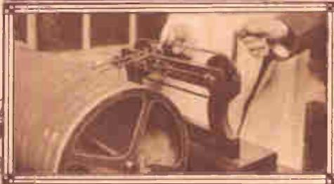
At the extreme left is shown another test for motormen. Here the driver is placed on a platform and a motion picture projected on a screen in front of him detailing the incidents along a route. The candidate's reactions to the various illustrations are noted. The photo at the left shows the Benet oscillograph for measuring the speed of motor nerve impulses in the hand and arm.
