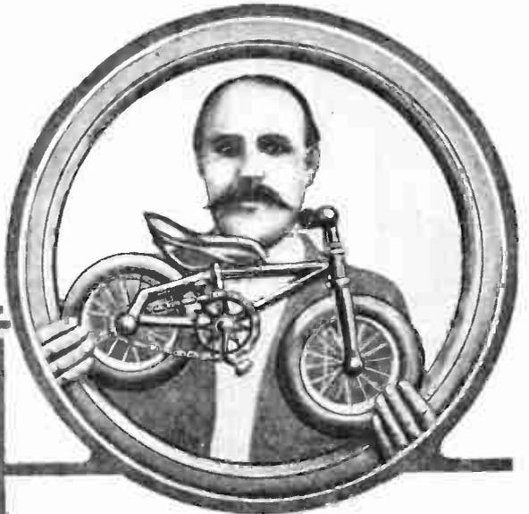
The miniature bicycle shown in the photograph above is perfect in every mechanical and functioning detail. This tiny bike was made for the performing monkey on the theatrical circuit. It is exactly twenty inches long, and will revolve in an ordinary twenty-eight inch bicycle rim. It is a treat to watch its tiny owner propel it on a table top.
