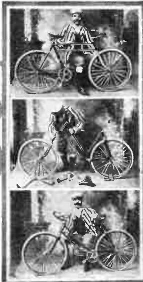
Above: The quick change bicycle which can be converted instantaneously into a truss frame for boys, and a drop frame for girls.
