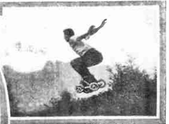
The German invention illustrated here has rubber-tired wheels about 5 inches in diameter. The weight of both skates is about seven and a half pounds.
