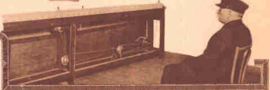
At the extreme left is shown another test for motormen. Here the driver is placed on a platform and a motion picture projected on a screen in front of him detailing the incidents along a route. The candidate's reactions to the various illustrations are noted. The photo at the left shows the Benet oscillograph for measuring the speed of motor nerve impulses in the hand and arm.
