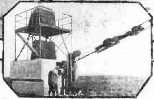
Above: Showing the immense area of ground occupied by the antenna system which is rigidly guyed and carefully anchored to large concrete blocks, by strain insulators.
