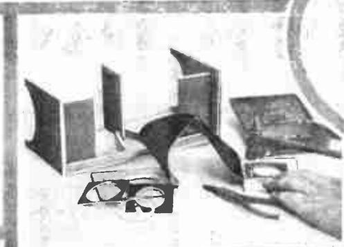
Four circles of cardboard are used as lens holders, and these are nailed in place, as shown above on cigar box slides. The cloth binding between prevents the eyes from glancing at the wrong picture. Photo at the left shows nailing the picture holder side in place.
