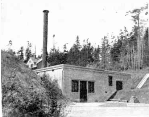
Power plant with engineer's and fireman's quarters in background. Earthworks are thrown up to the height of the roof around plant
