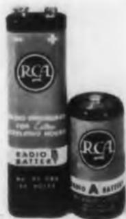
The VS086 45v alkaline-type "B" Battery weighs approximately 3 oz and measures 3-9/16" x 1-1/16" x 11/16" deep. It is intended for use in current personal portable radios designed to operate from a 45v "B" battery and a separate "A" cell.
