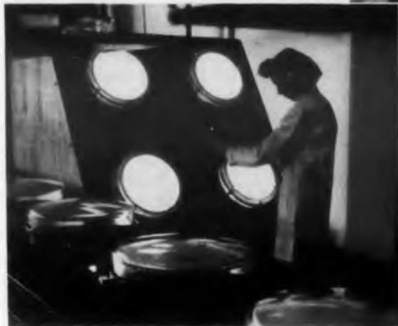
Unique photographic process, like photoengraving, uses aperture masks as negatives to print consecutively the red, green, and blue phosphor dots (250,000 of each) on CBS-Colortron screens.
