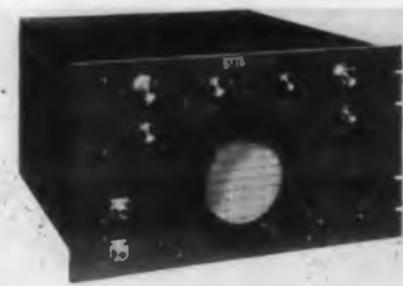
The Model 600 Cathode Ray Indicator is designed to utilize the high-writing-speed capabilities of the type 5XP cathode ray tube in applications too ad-
