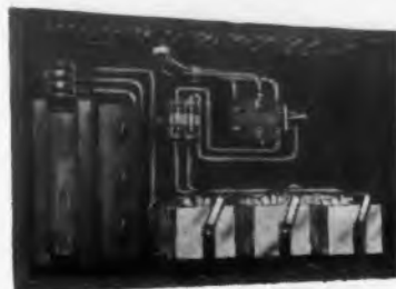
INSTALLATION AT TRIBOROUGH BRIDGE, 60 VOLTS OUTPUT, 45 AMPS. CONTINUOUS DUTY, OPERATING 24 HOURS A DAY, 365 DAYS A YEAR.
