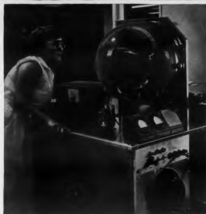
**Above:** metal parts for G-E micro-miniatures are fired in a high-vacuum furnace. Titanium is employed—this substance has the unique advantage of freeing virtually all its own gases when fired to 700 C. Result of using pre-fired titanium parts: there is no subsequent vacuum contamination from metal-liberated gases when tubes operate at high temperatures. Instead, titanium serves as a gas absorber!
