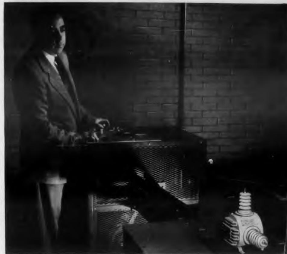
ONE OF MANY TESTS made on G-E oil-filled components is this six-hour vibration check.
