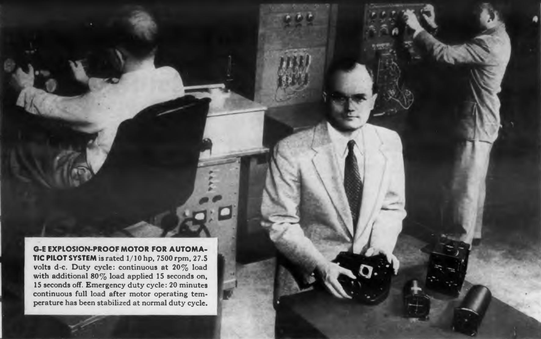
**G-E EXPLOSION-PROOF MOTOR FOR AUTOMATIC PILOT SYSTEM** is rated 1/10 hp, 7500 rpm, 27.5 volts d-c. Duty cycle: continuous at 20% load with additional 80% load applied 15 seconds on, 15 seconds off. Emergency duty cycle: 20 minutes continuous full load after motor operating temperature has been stabilized at normal duty cycle.
