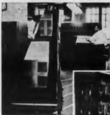
DASAC Push Button Control Center which uses Clare relays and stepping switches in automatic control of warehouse assorting system
