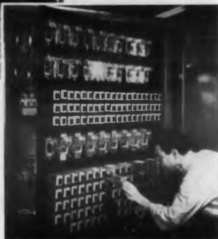
Rear view of panel shows Clare relays, provided with dust light covers, accessible for quick inspection and maintenance
